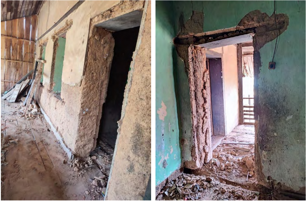
Plate 8 (a-c): Plaster-replacement around doorways and on walls, generally.
