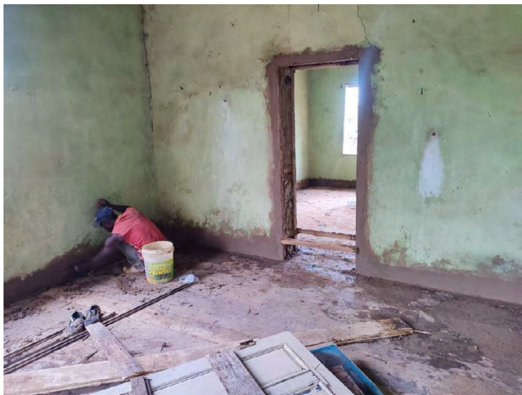
Plate 8 (a-c): Plaster-replacement around doorways and on walls, generally.
