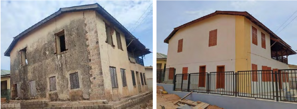
Plate 17 (a & b): Hinderer House; left flank/ approach façade. Note the restoration of two windows on the ground floor to doors.
