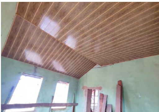
Plate 13 (a-c): Interior ceilings, after repairs. Note the use of PVC slats in b & c.
