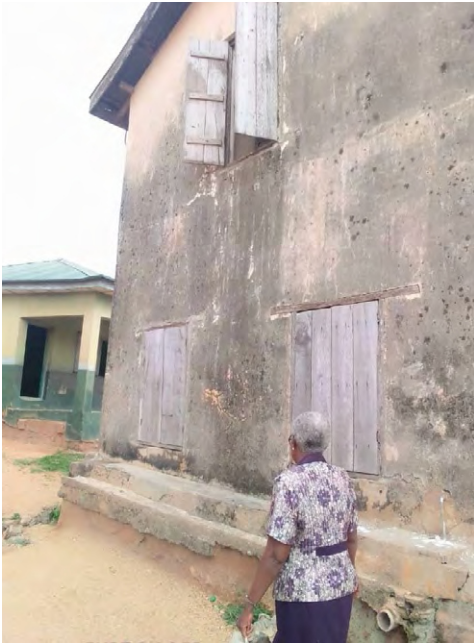
Plate 3 (a & b): Hinderer House – different wings, showing eroded building plinth & dilapidated windows.
