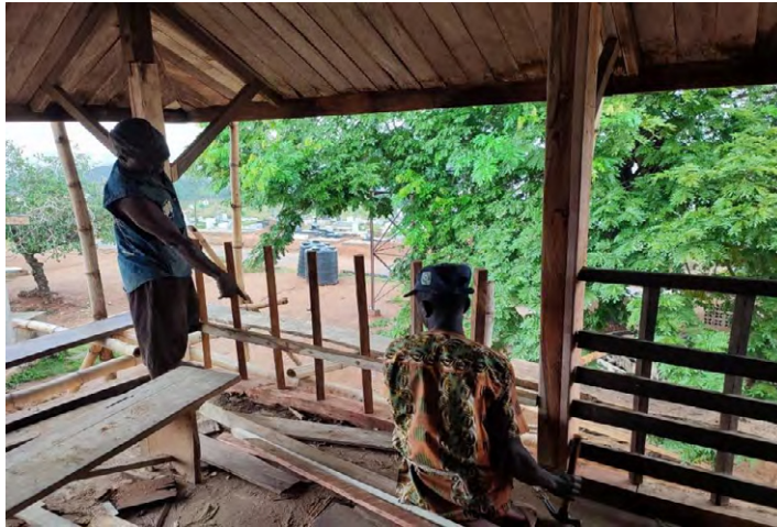
Plate 10: Replacement of defective timber posts and railings.
