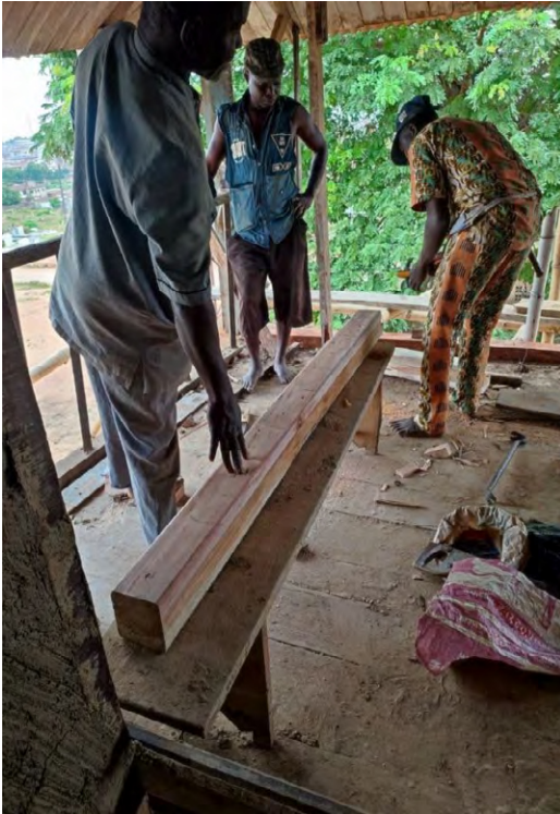
Plate 9 (a-b): Removal of defective timber posts & railings.
