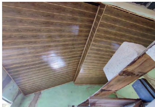
Plate 13 (a-c): Interior ceilings, after repairs. Note the use of PVC slats in b & c.
