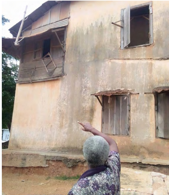
Plate 3 (a & b): Hinderer House – different wings, showing eroded building plinth & dilapidated windows.
