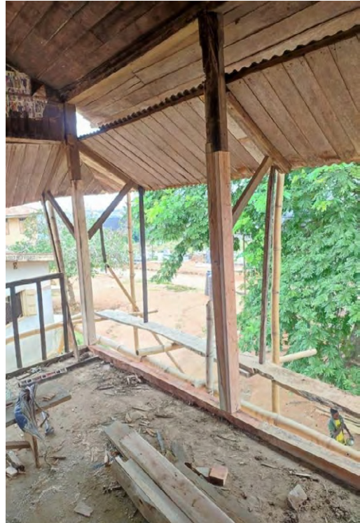
Plate 9 (a-b): Removal of defective timber posts & railings.
