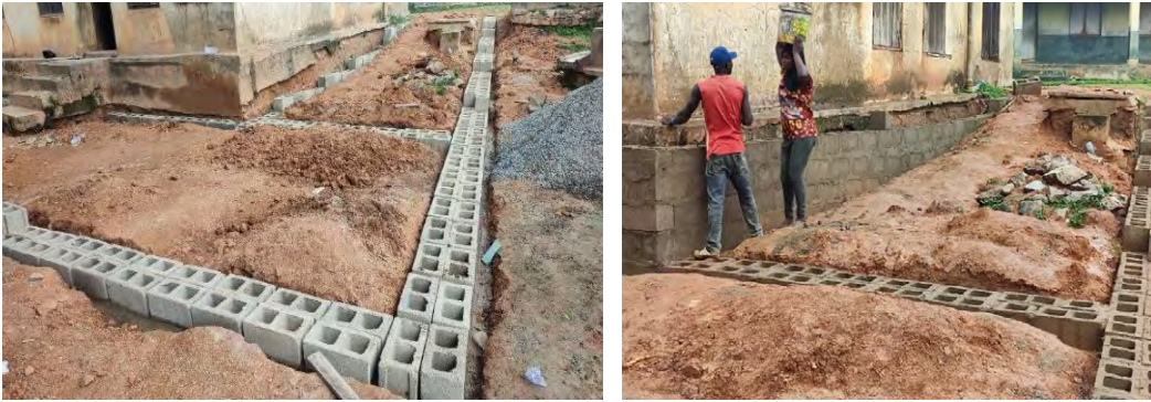
Plate 7 (a-d): External works – foundation consolidation: plinth/ retaining wall.
