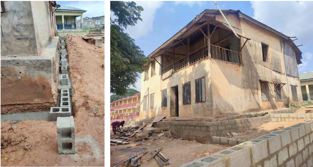
Plate 7 (a-d): External works – foundation consolidation: plinth/ retaining wall.
