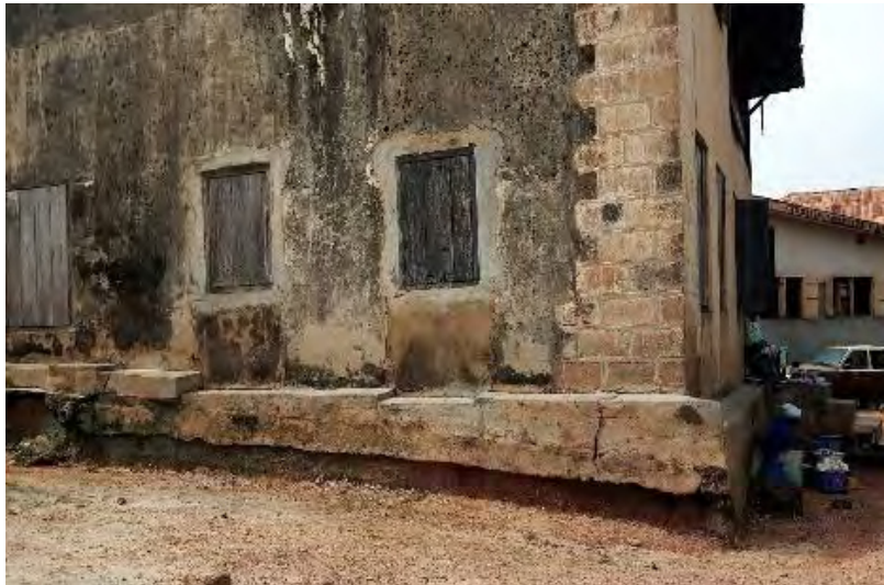
Plate 4: Building corner done in stone, accentuated by pointing in cement-plaster. Notice the eroded plinth, as well.
